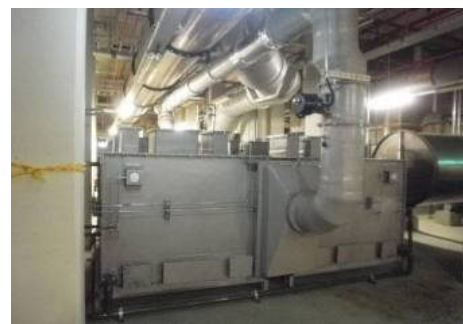
除臭常溫觸媒吸附塔 (Deodorization Catalyst Adsorber)
